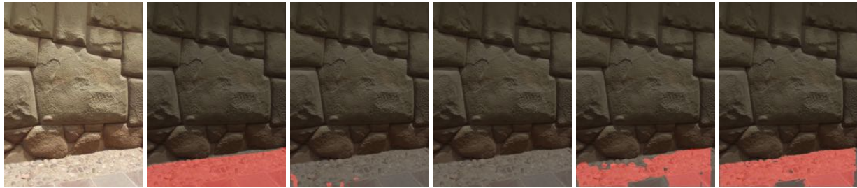
The ground below the wall.
